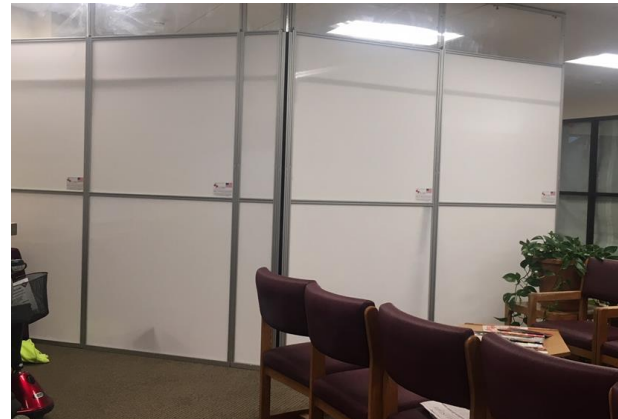
The view from the current waiting room. The crews are working behind these barriers to tie new and existing spaces together.
