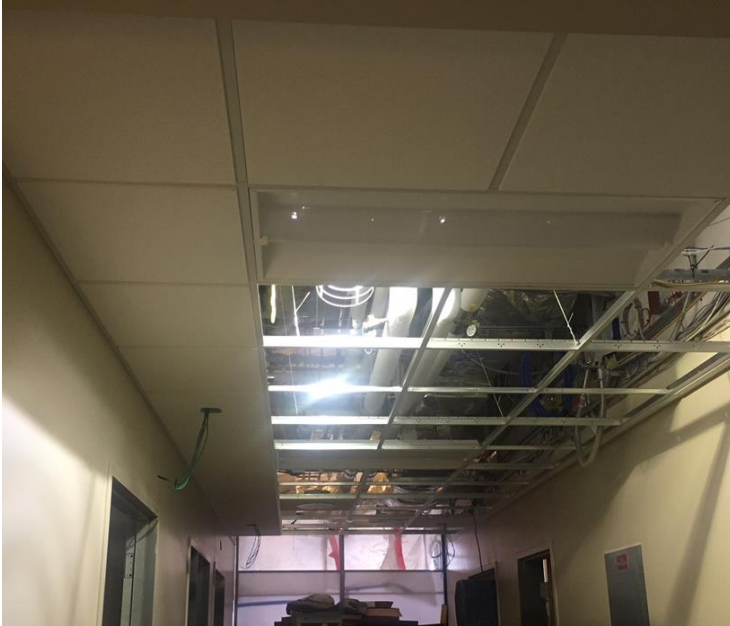
A ceiling is being added and finished up that leads into the new “Main Street” area at the end of the corridor.
