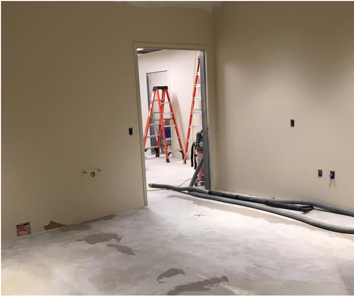
Floor prep is involved in each room before the actual flooring materials can be placed down. This helps ensure a flat floor.
