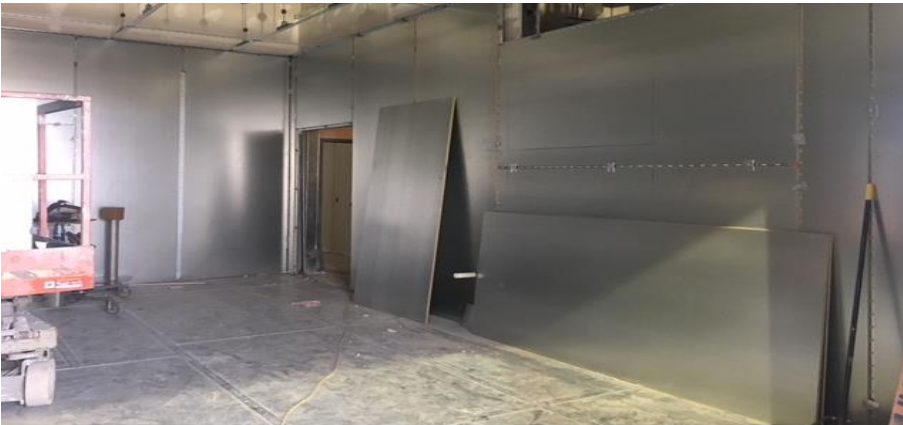
A special shielding is added to the walls, floors, and ceiling of the MRI room! This stops the magnetic force from traveling beyond the walls of that specific room.
