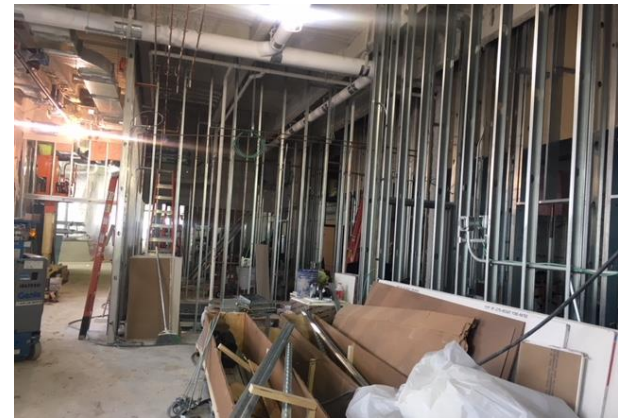
This framing currently outlines the new "Main Street" area that will feature a deli and seating.
