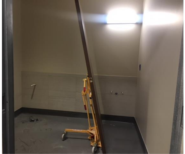
This cart, sometimes called a door jack, helps the carpenters install the doors quickly and correctly. Doors are currently being installed in the new Imaging area.
