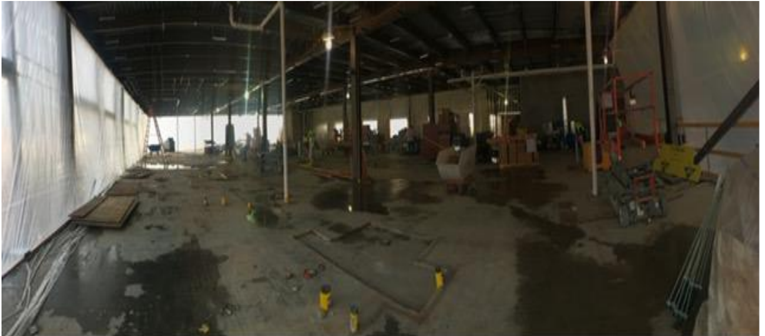
The overall view of the upper level portion of the new addition. The cut out shape in the floor towards the middle of the picture outlines where the bathrooms will be in each of the rooms. Soon walls will be added around each area to help define the space.
