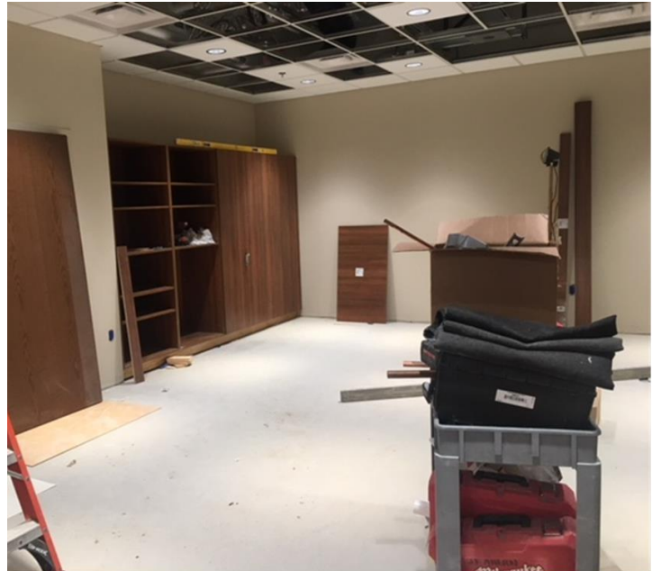
Casework is currently being installed in the Imaging area.
