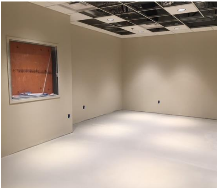
In certain Imaging area rooms, the entire floor in the room is leveled to prepare for the new equipment being installed.
