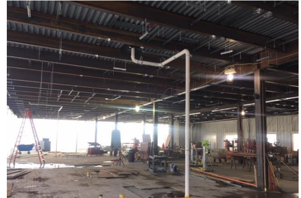
The upper level of the new addition is coming along quickly. Soon this area will be fireproofed.
