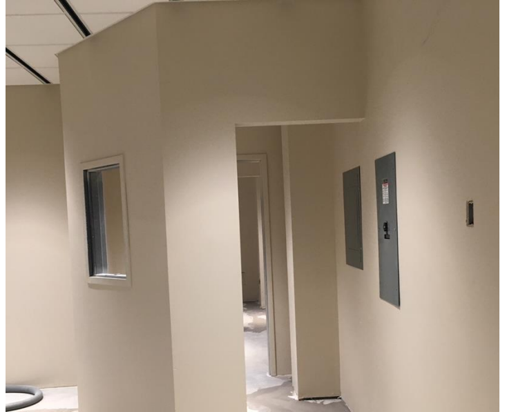
The new control room connects the Fluoro room with the X Ray room!
